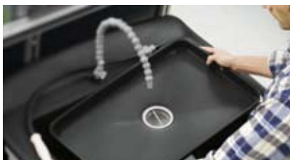
Place sink base with drain in position
